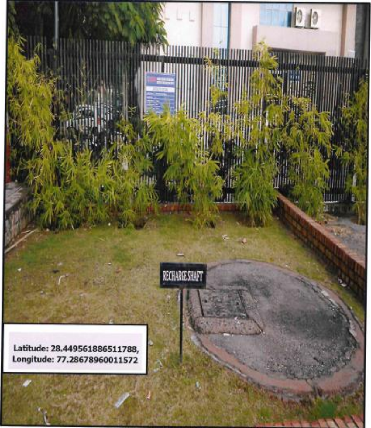
Rain Water Harvesting Ground Water Recharge Shaft T Block
