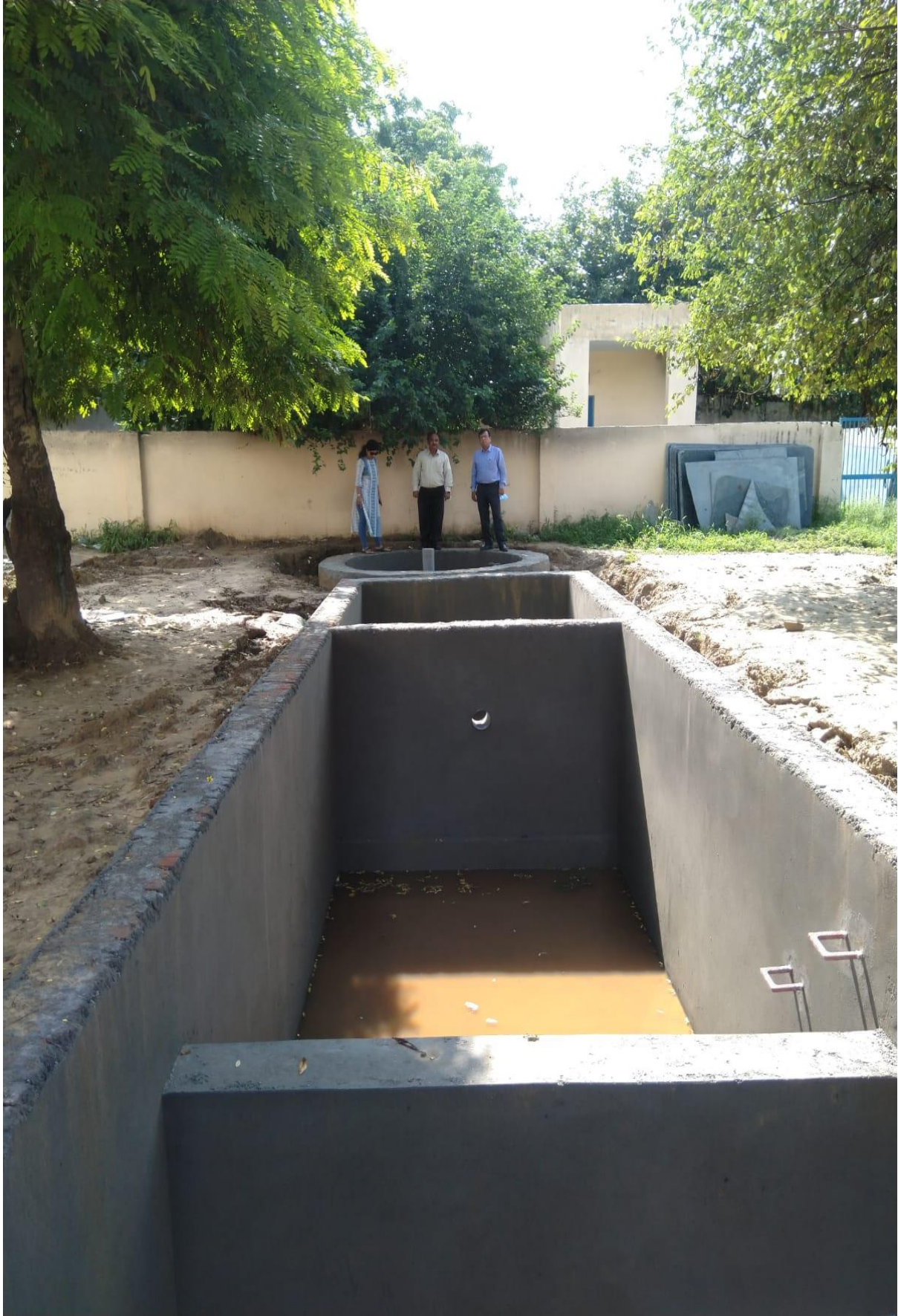
Constructed Structure at Officer's Colony, Sector 15A of Faridabad City of Haryana State of India
