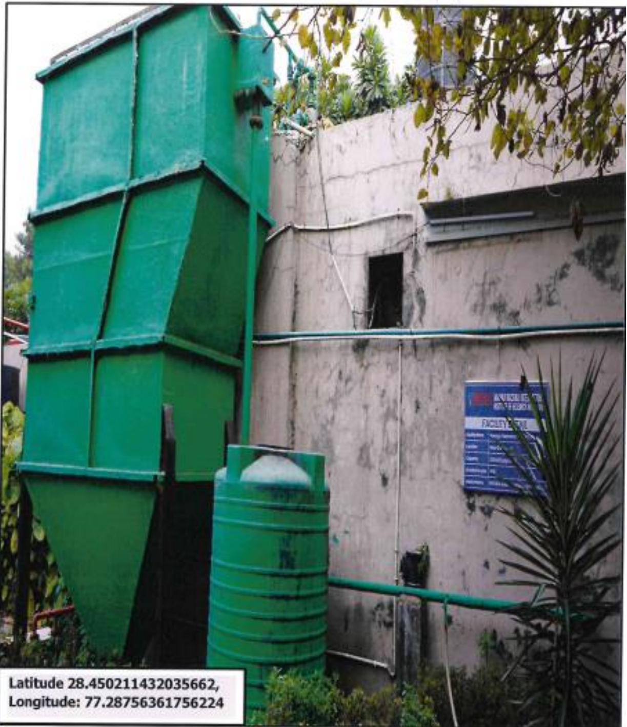
Sludge Tanks ,Sewage Treatment Plant
