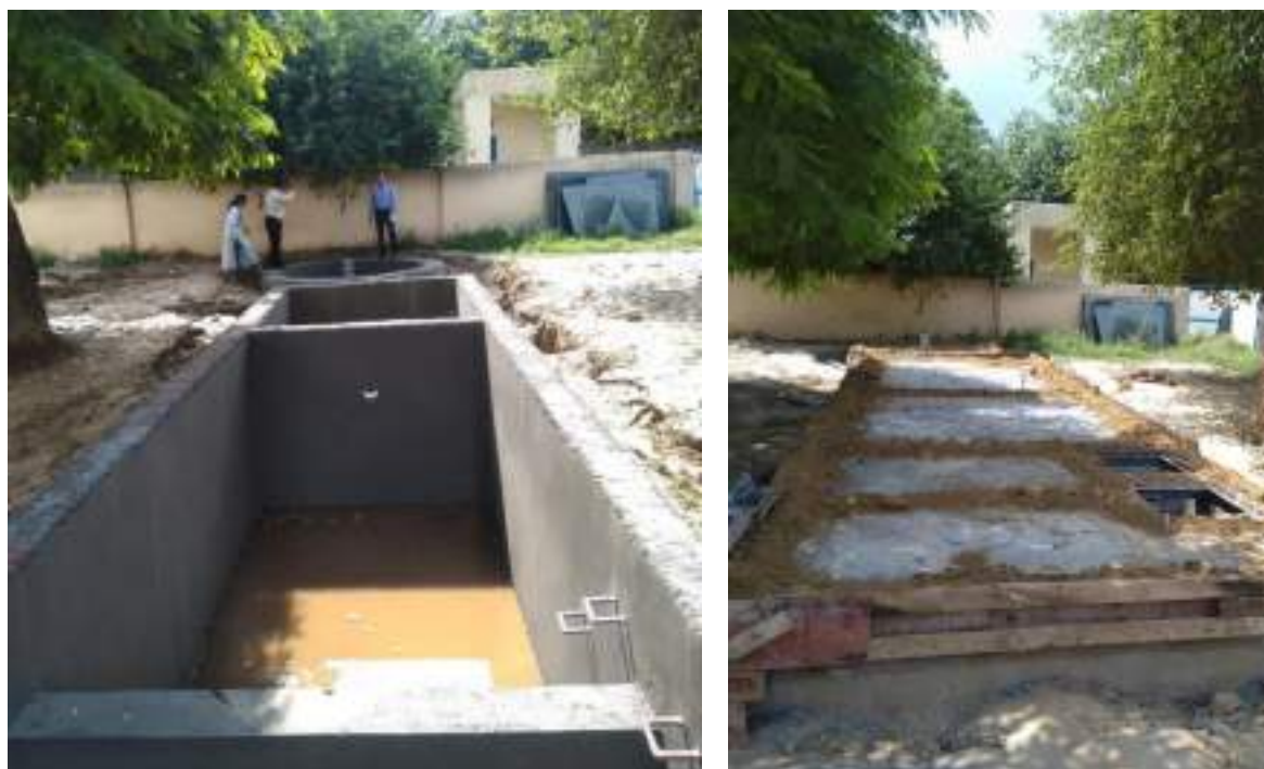
Fig 10. Photographs of constructed desilting and coagulation chambers and dug cum recharge well at Officers Colony.
