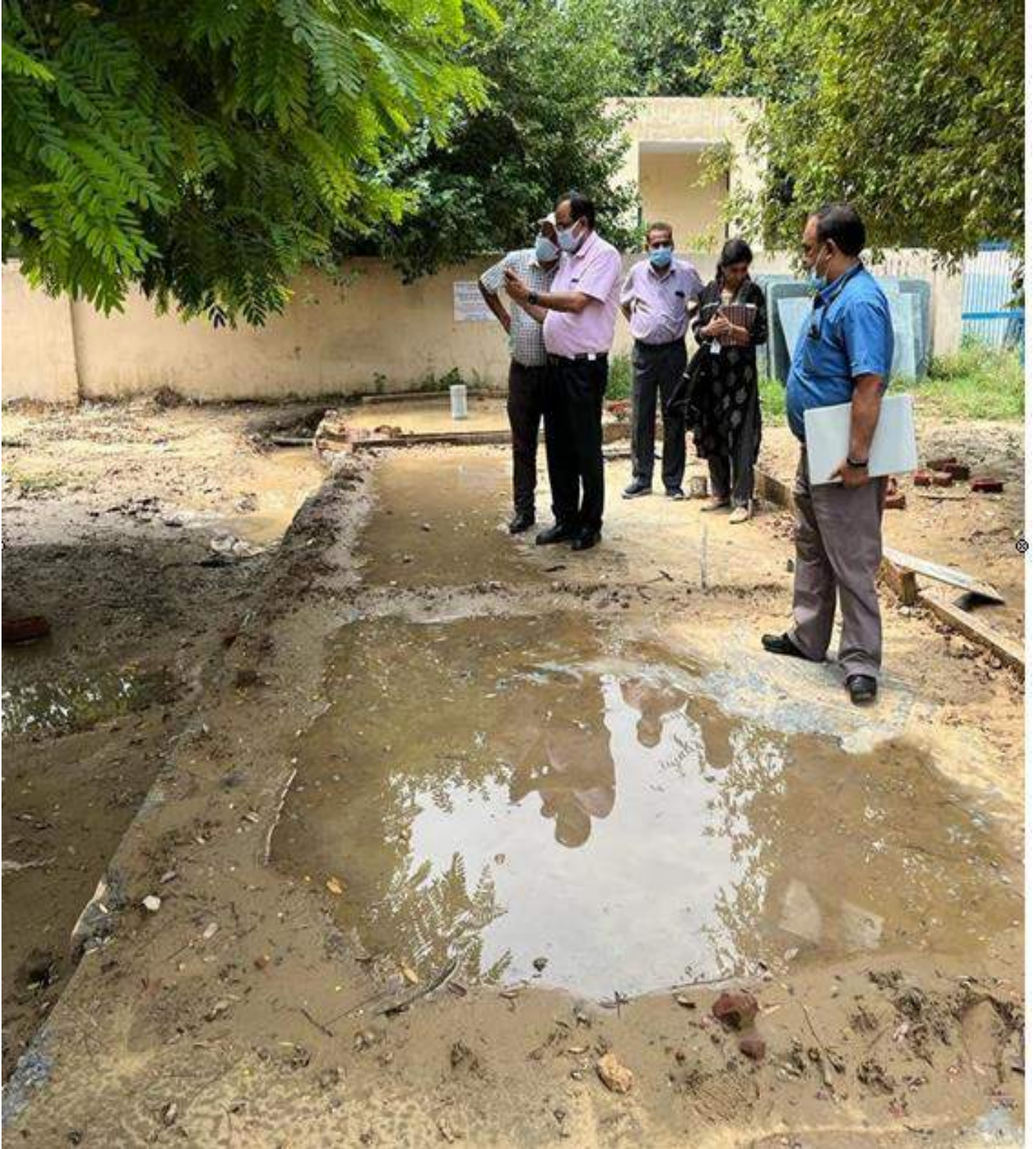
Inspection of site - Officer's Colony, Sector 15A of Faridabad City of Haryana State of India
