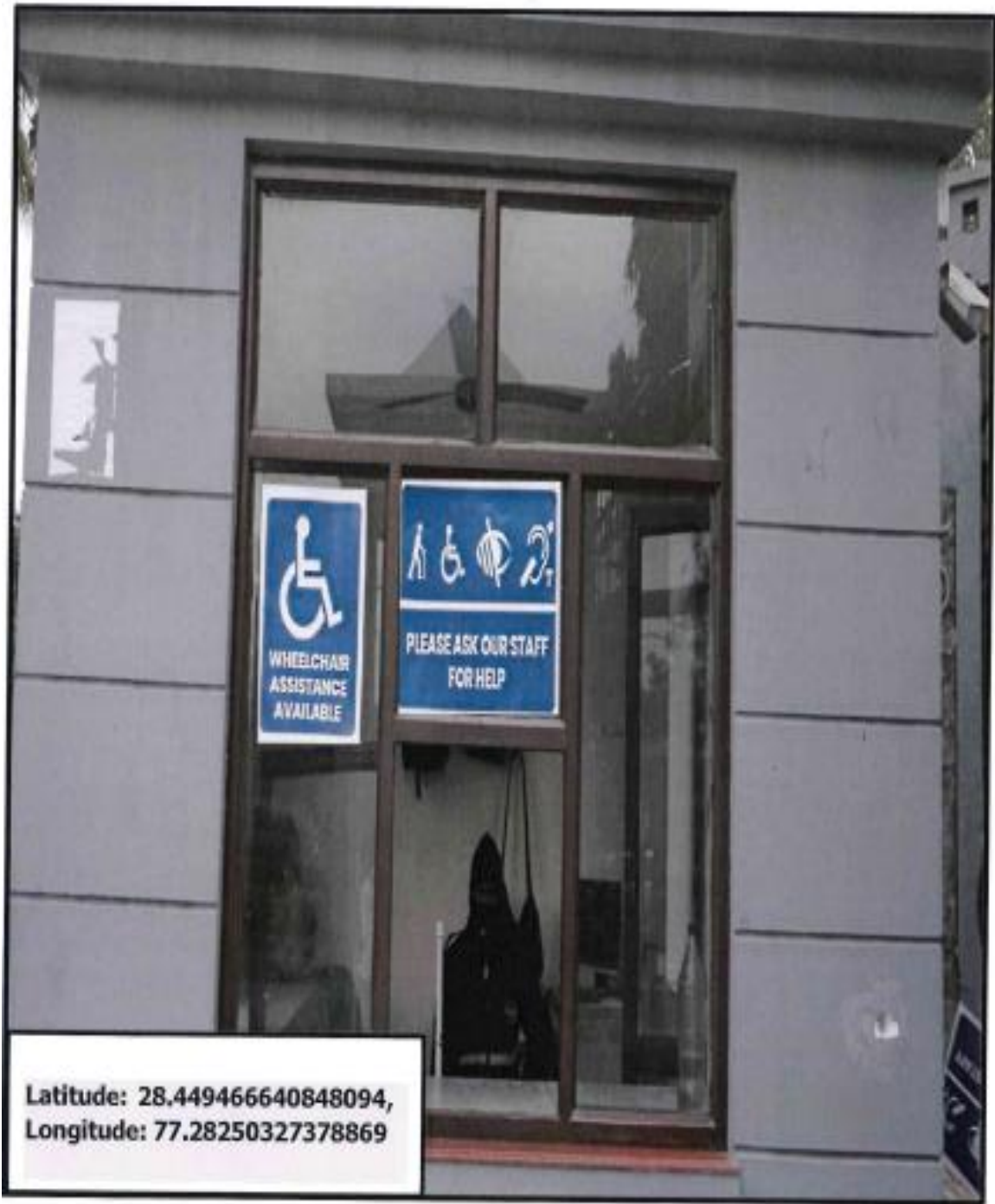
Disability Support Office (with availability of Mechanized Equipments)
