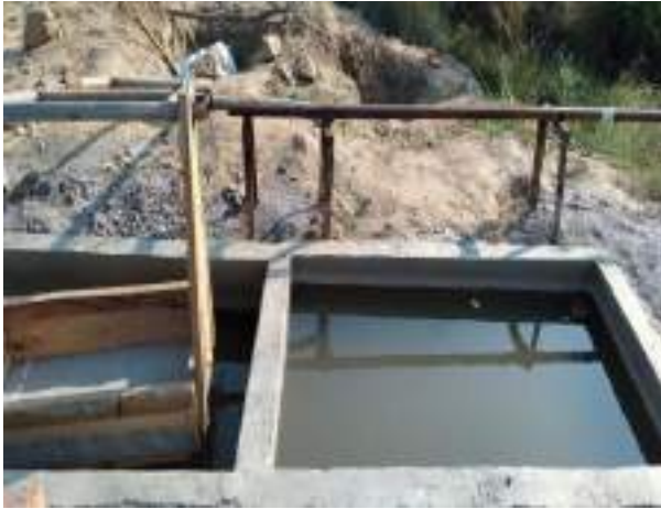
Fig: 9.2 Showing two settling ponds for collection of mine discharge
