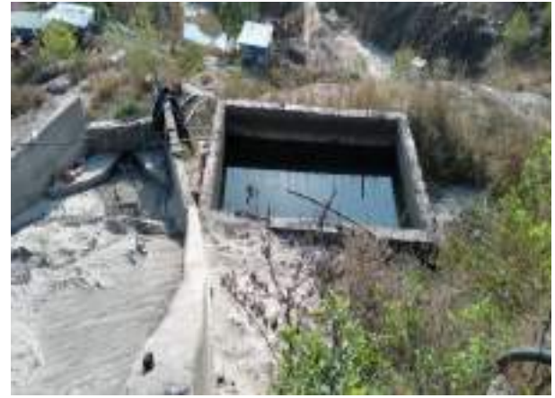
Fig: 9.2 Showing two settling ponds for collection of mine discharge
