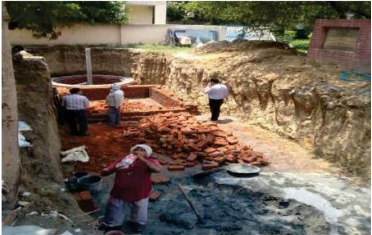
Construction of Structures for Co-solving of Water Logging and Ground Water Depletion Issues in Officer's Colony, Sector 15A of Faridabad City of Haryana State of India
