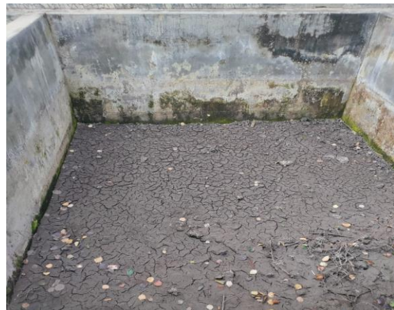
Sludge drying bed
