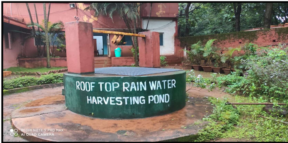
Fig-7.4: Roof Top Rainwater Harvesting in Lease area.
