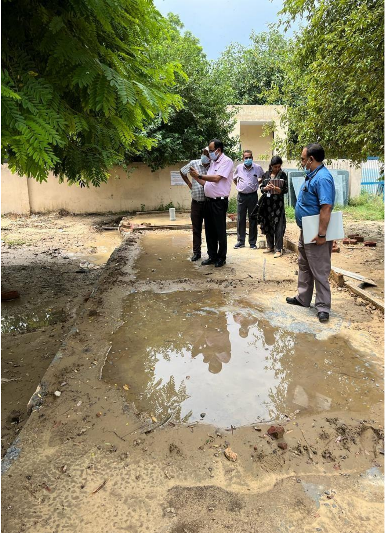
Inspection of site - Officer's Colony, Sector 15A of Faridabad City of Haryana State of India
