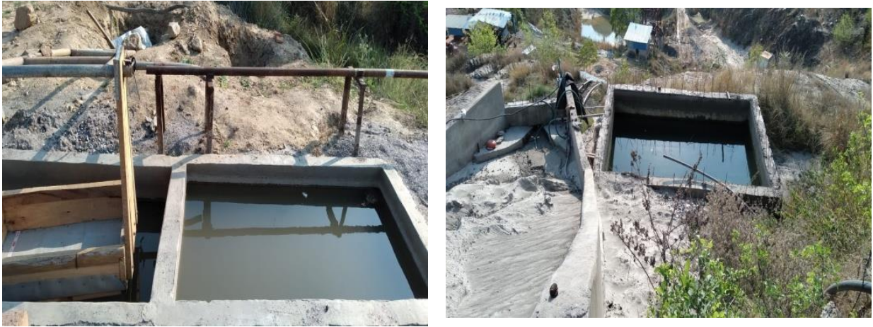
Fig: 9.2 Showing two settling ponds for collection of mine discharge
