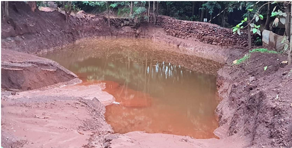
Fig-7.3: Rainwater Harvesting Pond
