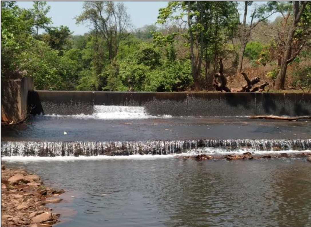
Fig 2.7: Existing water harvesting structure in Buffer Zone
