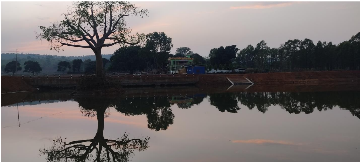
Fig 2.8: Existing rainwater harvesting pond and mine pit storage tank in Buffer Zone.
