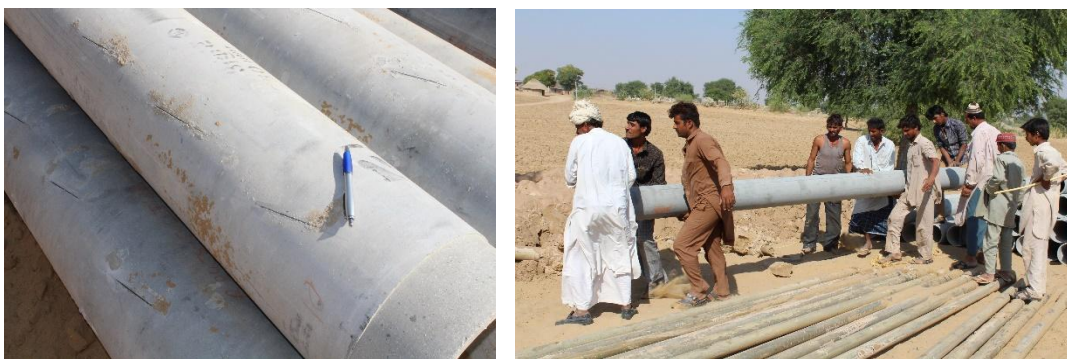
Fig 10.4: Casing Pipe used in Barmer for Tube well construction.
