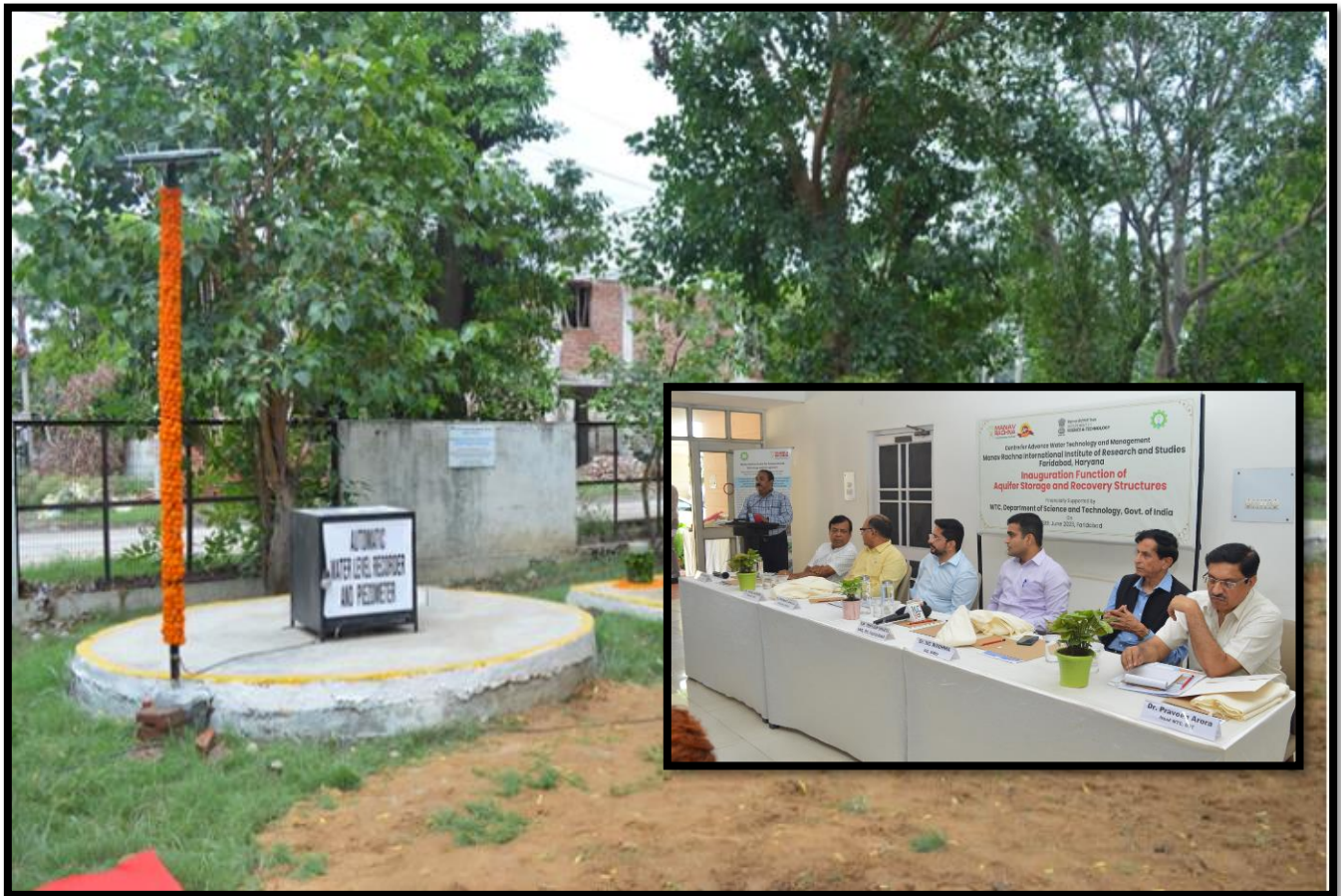
Fig Actual pictures of site at Sector 16A B&R Faridabad, before and after construction of ARS System and inauguration event.
