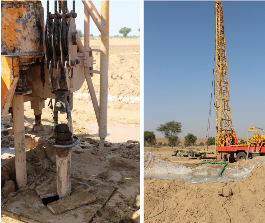
Fig 10.1: Construction of a new tube well by rotary drilling rig
