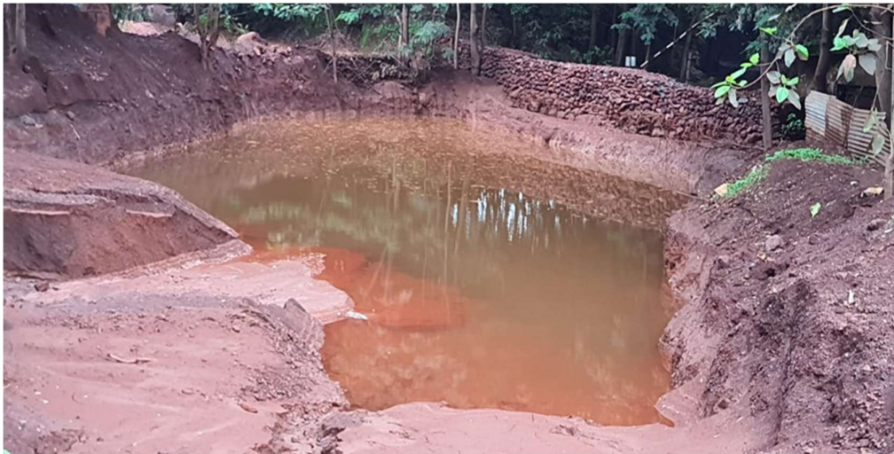
Fig-7.3: Rainwater Harvesting Pond
