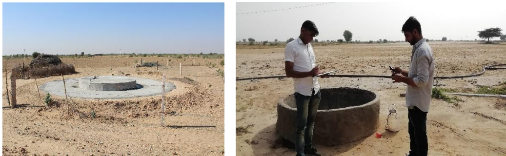
Fig 10.5: Rainwater harvesting structure as Taanka in the Barmer area.
