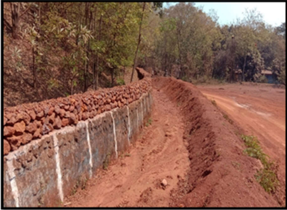
Fig 7.1: Retaining Walls and Garland Drain in Mining area
