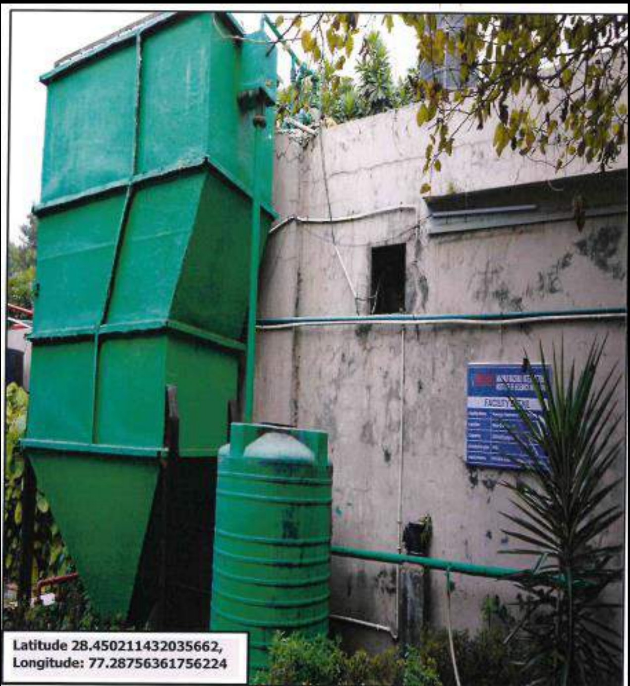
Sludge Tanks ,Sewage Treatment Plant
