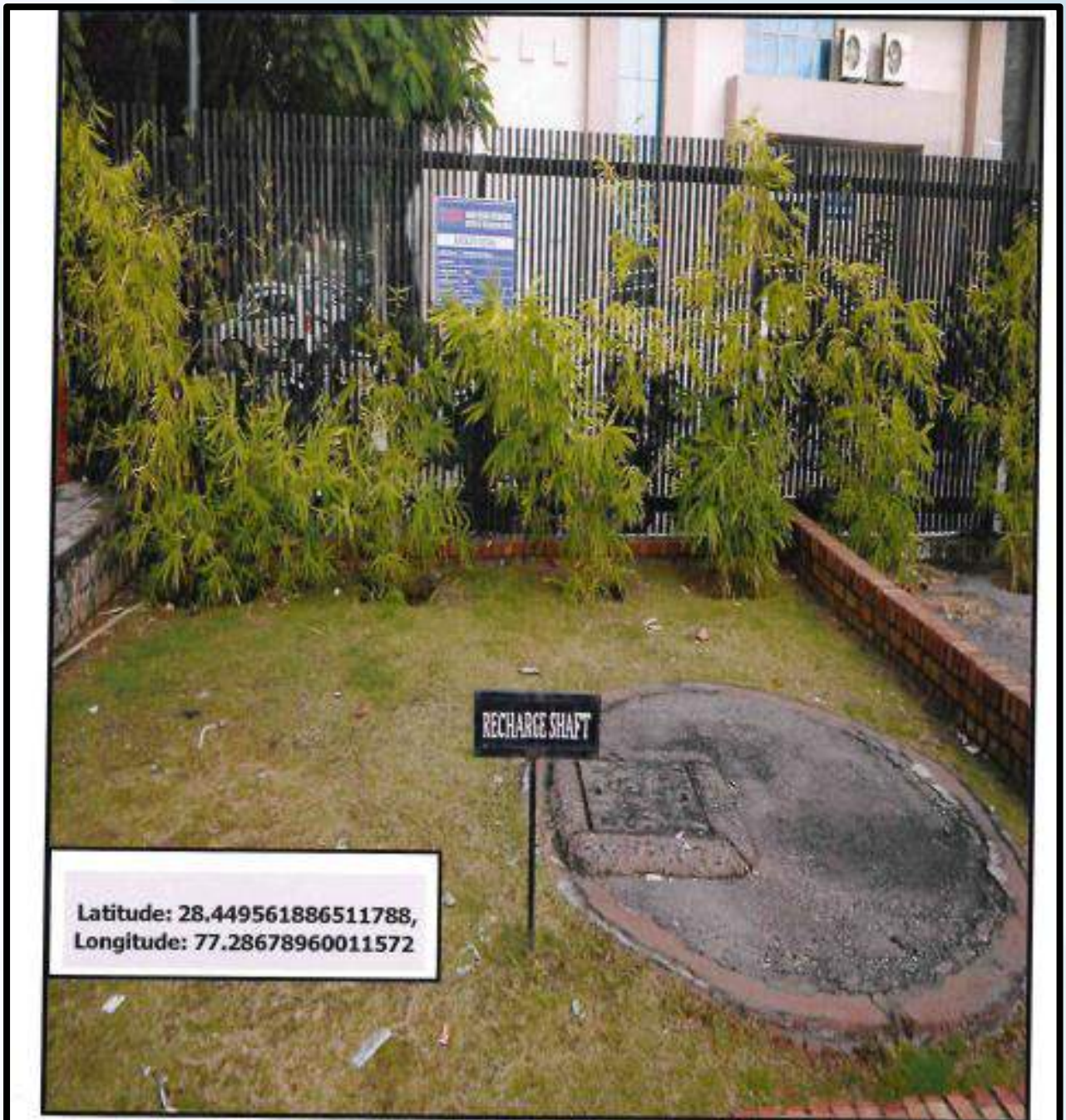
Rain Water Harvesting Ground Water Recharge Shaft T Block
